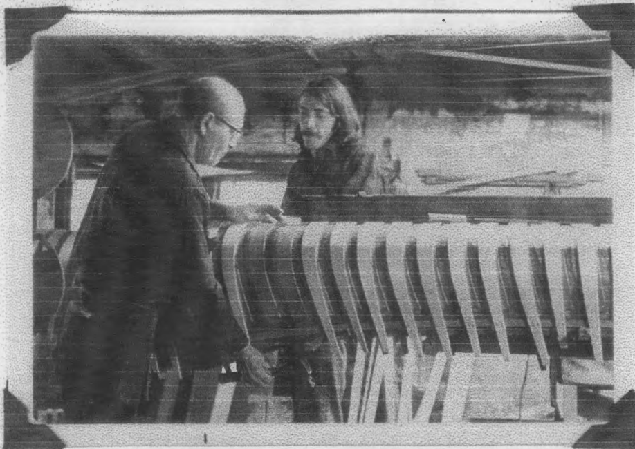
George Fletcher, left, and helper applying steamed ribs to the mold. Note iron bands on the mold, also the brace bolted to hold the ribs in place. Examining closely, one can see the notched inside keel and the inner gunwales.
