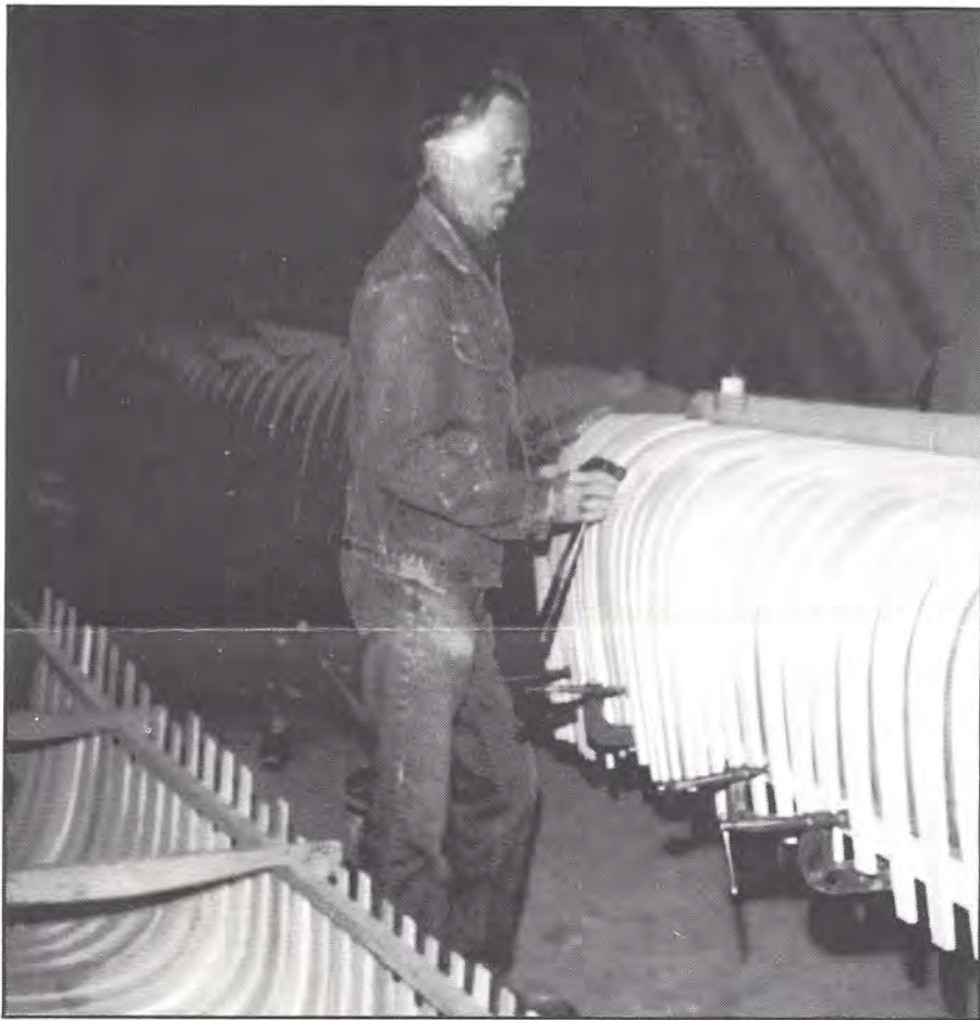
Carl Jones inspects the ribbing of a new canoe; the next step is planking.
